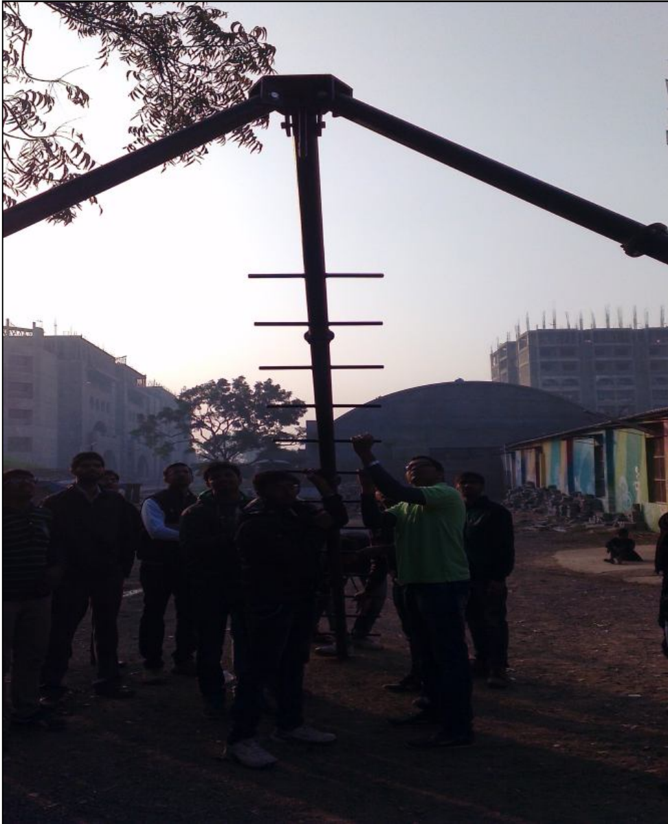
Assemble the SPT Setup
